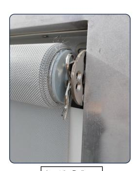
Insert the R-clip locking pin in place
