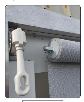
Inserting the square end into the gearbox
