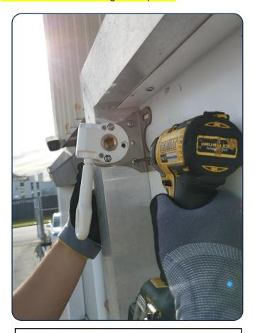
Screwing in the Gearbox bracket – Take note: the angle of the crank
