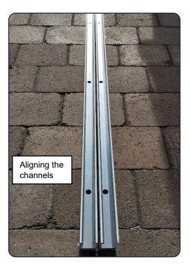
Ensure the **channels** are oriented the same way (Align the holes on both channels so that they are in the same location on each side) then proceed to mark out and cut the side channel down to size.
