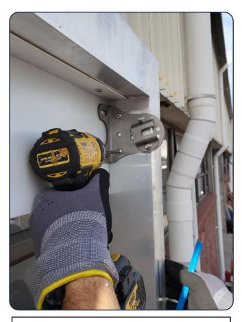
Screwing in the Pin plate bracket – Take note: the angle of the opening of the plate
